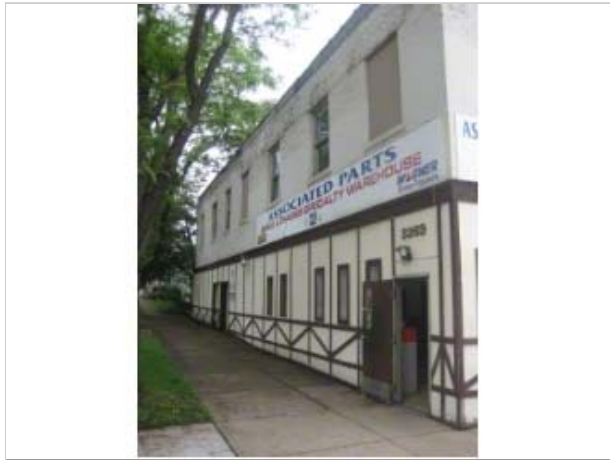
Associated Parts Store & Residential Apartments
